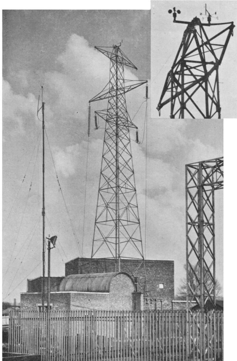
*Wind vane and anemometer topping the 120ft tower at Forrest's laboratory (Forrest, 1951)*
